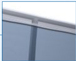
outside: fabric skin with spandex sleeve
